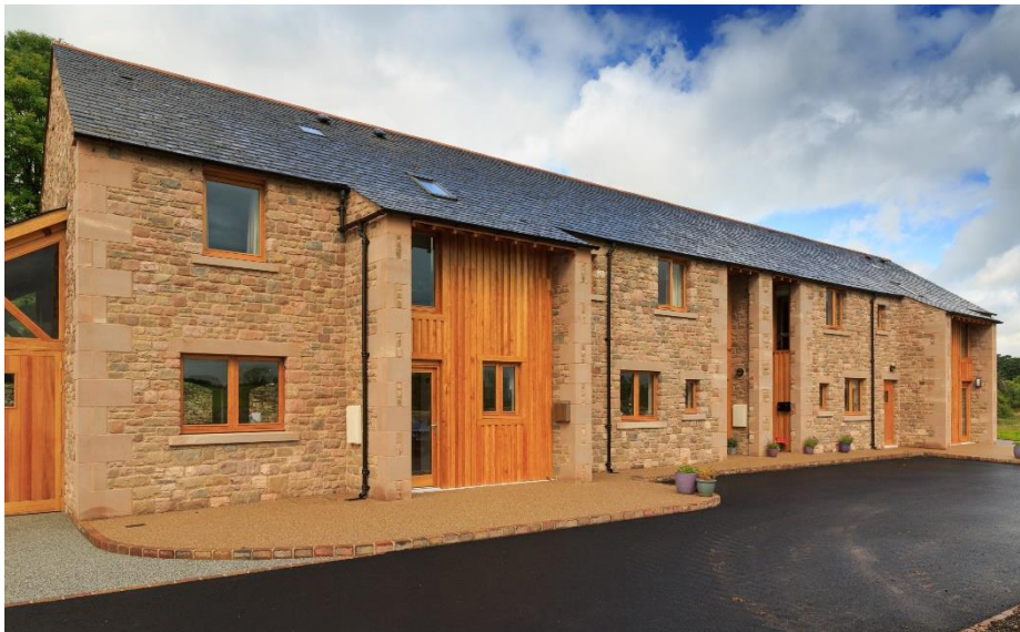
Wattscliffe quoins and surrounds used on a new development at Greystoke
