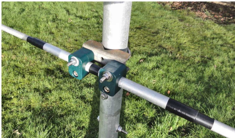
Figure 3: Construction of the two new elements.
