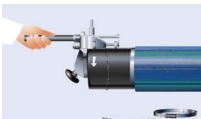
Fig 7-19: Removal of the oxide layer using a rotary scraper
