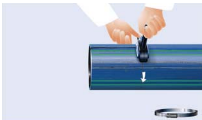
Fig 7-17: Removal of the protective coating with the egeplast M10 peeling tool
