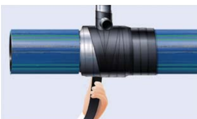
Fig 7-56: Wrapping the tapping fitting with Densolen Tape AS 40
