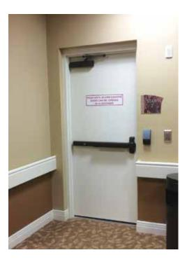
The Von Duprin CHEXIT delayed egress device provided the facility manager with a security and safety solution tailored for a memory care environment.
