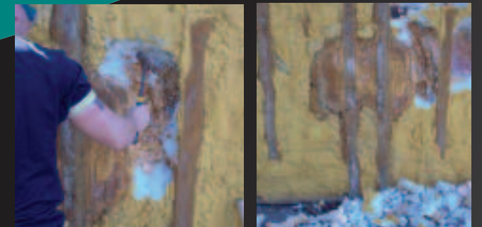
Servicing a Foamed Filled Spa
