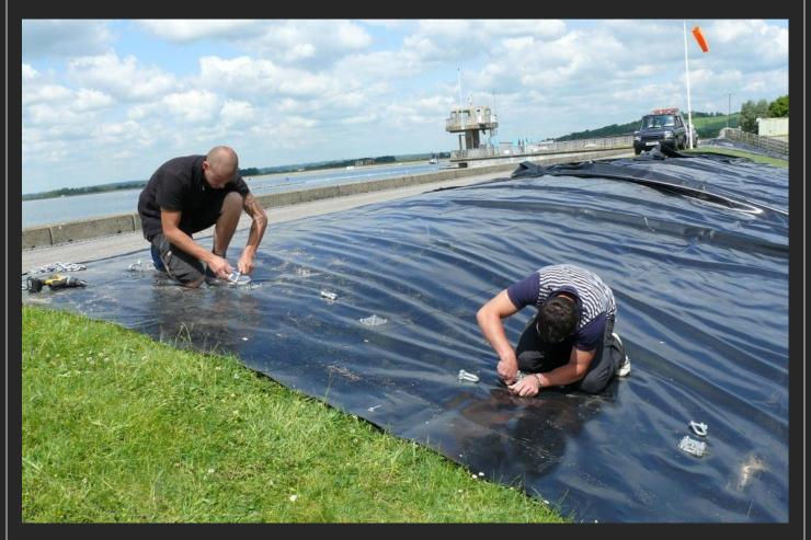
Almost 2000m<sup>2</sup> of baffles and curtains, along with almost 10,000m<sup>2</sup> of accretion materials for biological attachment were fabricated and installed within and below the 210m<sup>2</sup> floating system.
