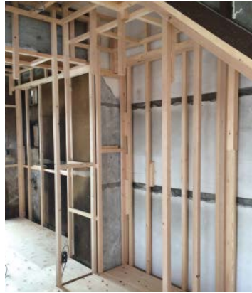
壁面の断熱施工例 before after
