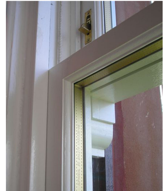
Top left: 'Slimline' double glazing in historic frame and retention of original ironmongery
