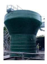
8m diameter x 9m tall clarifier with 6o degree cone supported on an integrally wound support skirt. Believed to be the largest one piece, free standing tank of its type in Europe – Dwr Cymru/Welsh Water, Brecon.
