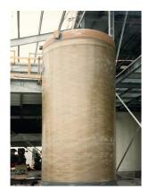
One of the 36 process vessels ranging from 1.2m to 4.5m diameter for a wide range of difficult chemicals which required linings of Isopthalic, Bisphenol, Vinyl ester and Furane resins – Conteka Catalyst plant, Delfzijl, Netherlands.
