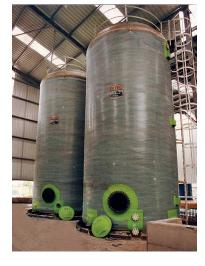
2 x 100m3 Industrial Waste Process Tanks handling mostly sulphuric acid with solvent traces. The operator reports that they are still performing satisfactorily after 20 years of service
