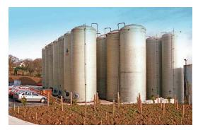
36 x 136m3 cider fermentation tanks with sludge settlement facility - Inches Cider, Devon
