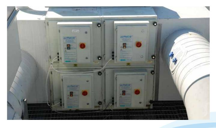
4 ESP Units Stacked in modular formation with a double pass
