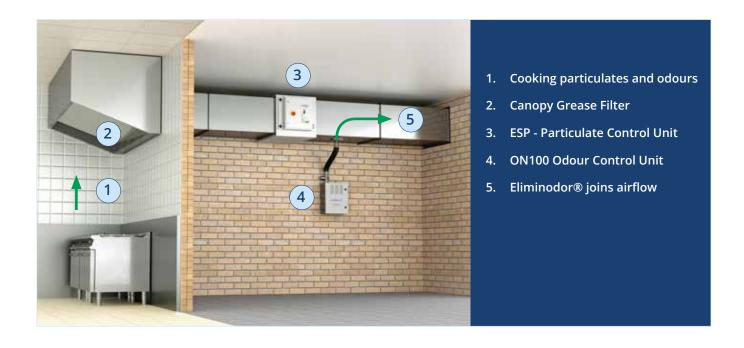
Once the airstream in the exhaust duct has had the majority of the particulates removed by one of our ESP units the gaseous phase or malodour can then be treated by the ON 100.
