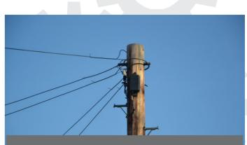
Pole Step, Ring Pole Head Dropwire and Clamp Dropwires on Telegraph Pole
