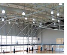
Sedona fabric duct with Comfort-Flow air dispersion and linear vents manufactured by DuctSox, Dubuque, Iowa, helped cut both material and installation costs. Gray 56-inch-diameter fabric duct distributes dry, conditioned air along a wall of exterior windows and three 36-inch-diameter ceiling-hung branches span the entire width of the pool surface. A
