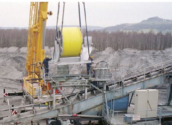
The experts at Conductix-Wampfler assist customers from planning through pre-assembly right up to the on-site installation - anywhere in the world
