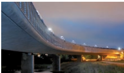
Lautrupsbach-Viaduct with Advance Bridge
