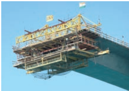
Cantilever carriage, Abu Dhabi
