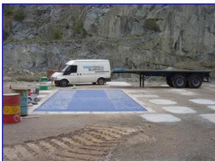
Pit mounted weighbridges are flush with the ground. As a result they pose no restrictions to vehicles and are therefore particularly useful at sites where vehicle flow can be in multiple directions. Most earlier mechanical weighbridges were installed in pits so when they are upgraded or replaced the new pit mounted weighbridges provide a very cost effective answer.
