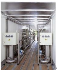
Maintenance is minimal with RO and UF elements typically lasting between 5 and 7 years depending on water source quality. Séon IFC uses standard coagulants and sterilising additives. The majority of component cleaning is automated by the system. Electronic systems monitor for faults and when low on additives and inform the user with the simple Siemens display.
