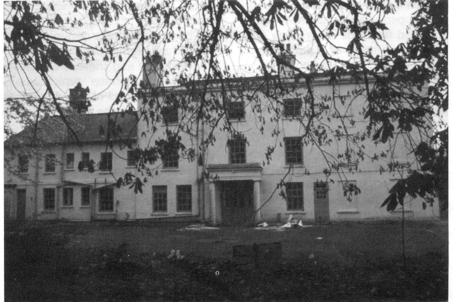
Harefield House, a Grade II listed building awaiting renovation
