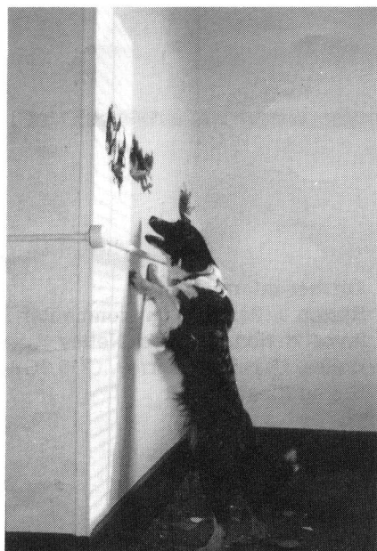
A Rothound indicates the presence of dry rot activity
