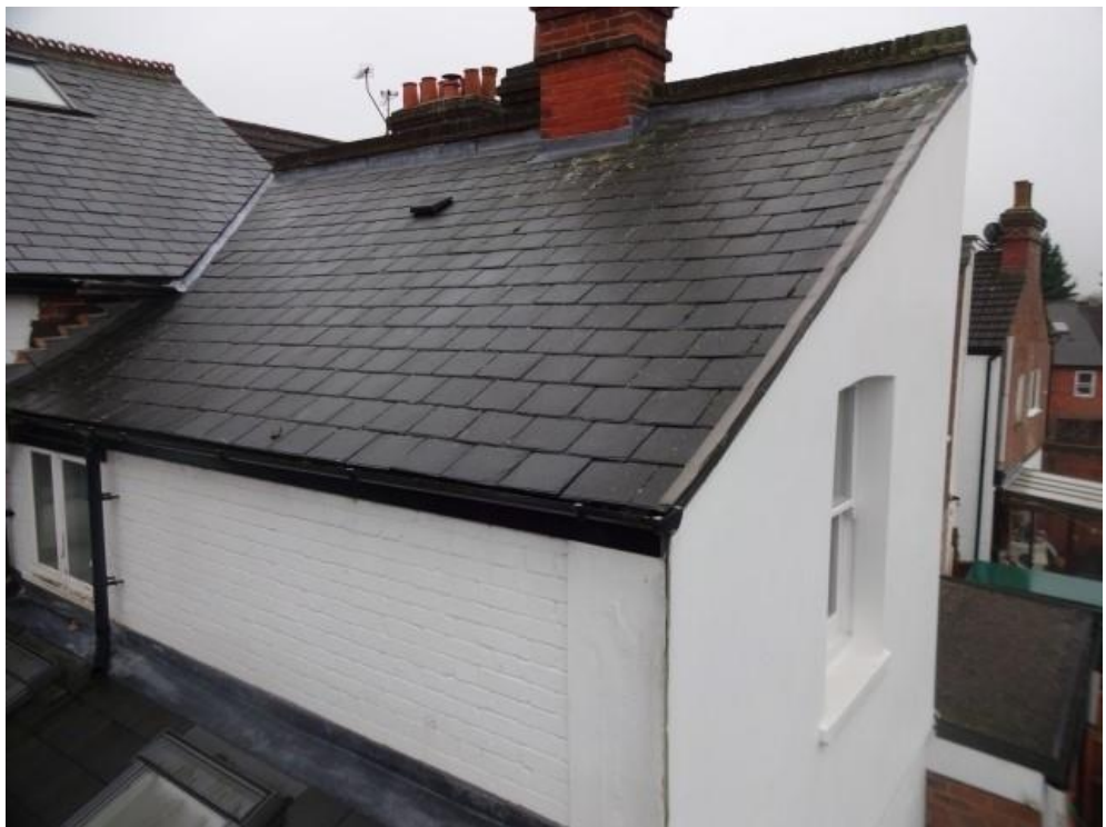
Roof over bathroom bedroom 3
