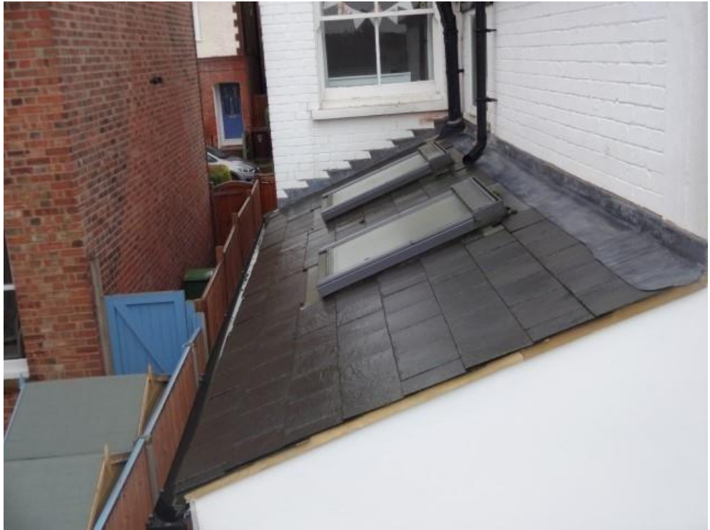
Roof over kitchen
