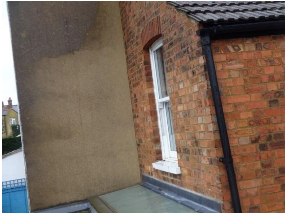
Next door in relation to rear bedroom 3 external wall
