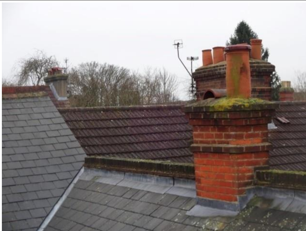
Rear redundant chimney stack
