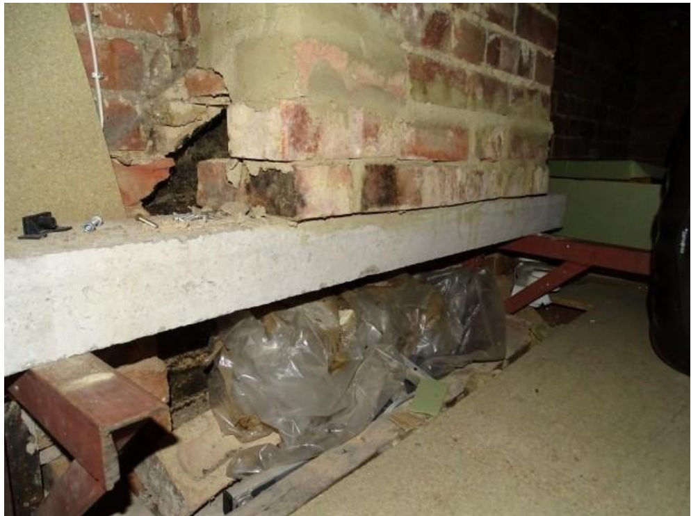
Chimney stack supported in loft
