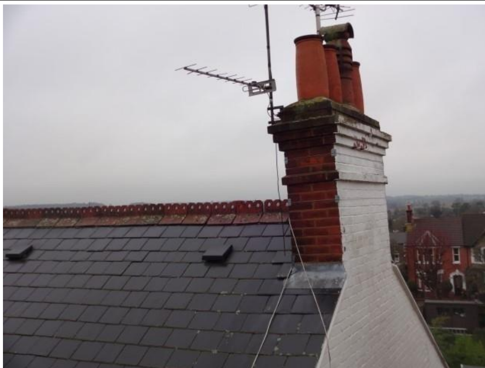
Front chimney stack
