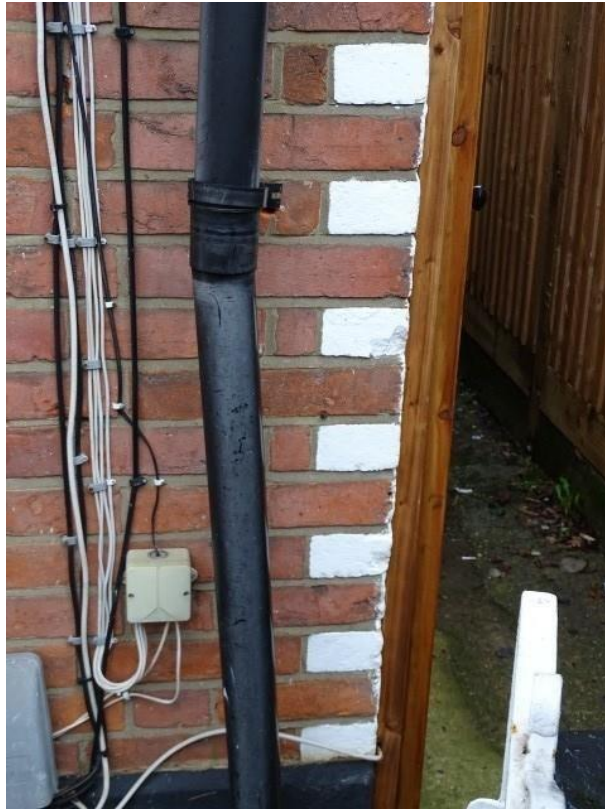
Front gutter down pipe
