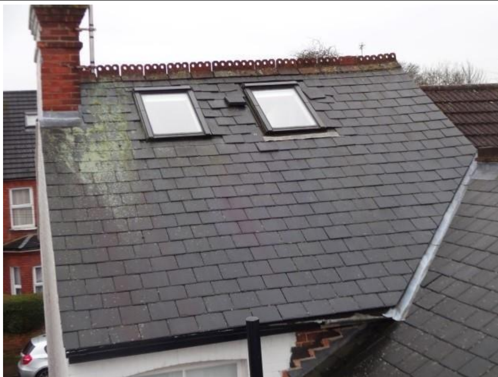
Roof over bedroom 2
