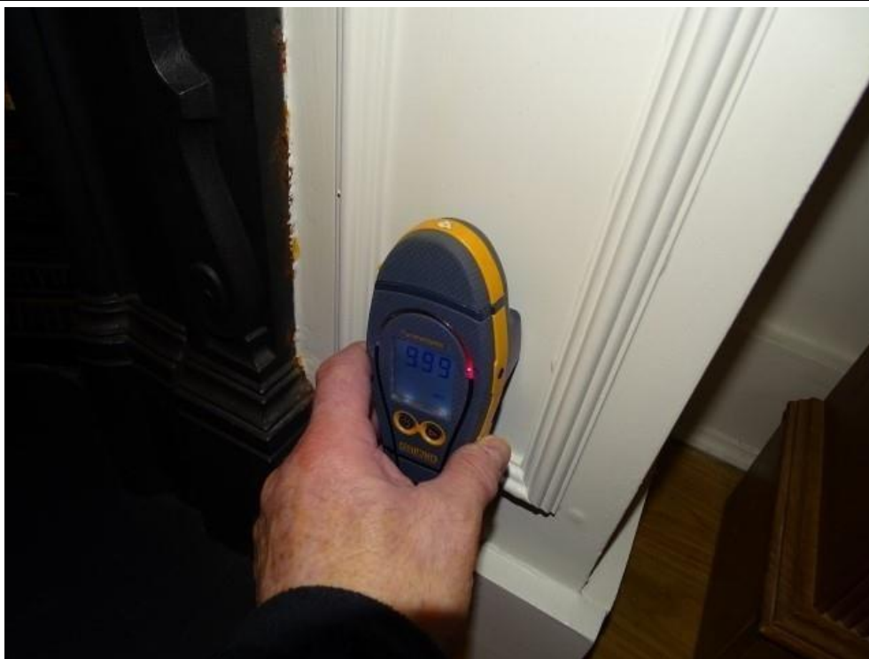
Chimney breast in dining room at low level
