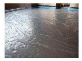
(c) Tape the 500 gauge membrane to the plastic skirt of the edging strip.
