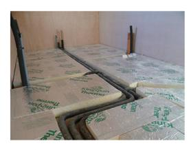
(b) Fill any voids around the pipes with dried sand and level off, then place the 2<sup>nd</sup> layer of insulation over the 1<sup>st</sup> layer, ensuring it remains flat, with no rocking.
