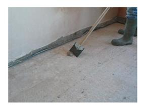
(b) Brush the sub floor, leaving a flat clean surface, on which to place the insulation.
