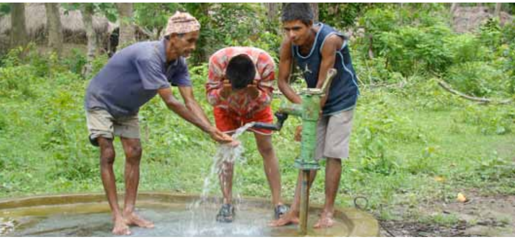
A water pump installed as part of the project
