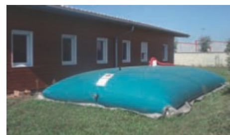
25 m 3 external rainwater recovery
