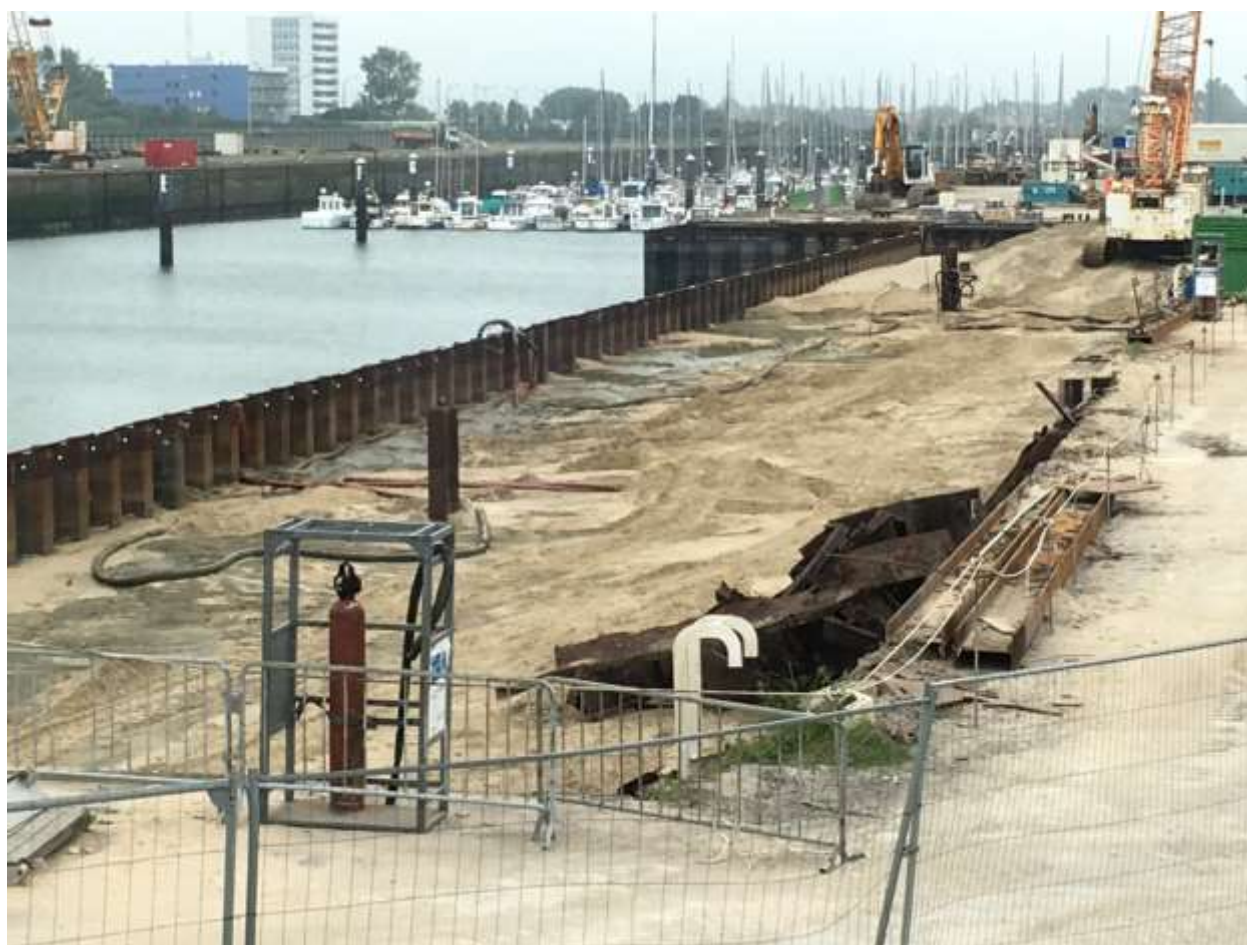
New infilling of northern part of Marina
