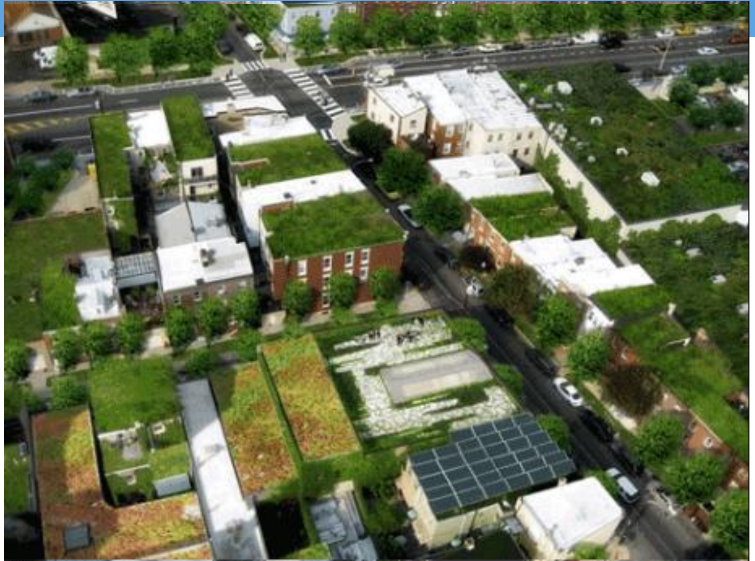
Green Roof Intro BEC St. Louis
