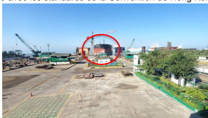
Chantier PHP. © Md. Zahirul Islam
