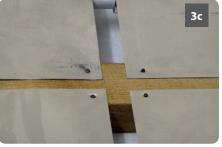
Wearing safety gloves due to sharp edges lift the first spreader plate into place measuring 250mm from the wall **(4a)** and fix the spreader plate along the top of the joists using staples, nails or screws ensuring they are flush fitting **(4b/c)**. Allow a 15mm expansion gap between each plate. A good tip is to press a short length of pipe into the pipe channel to help line up the plates before fixing in place **(4d)**.
