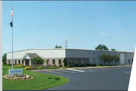
ELCo Enterprises headquarters in Jackson, Michigan
