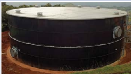
Trough Deck Roof
