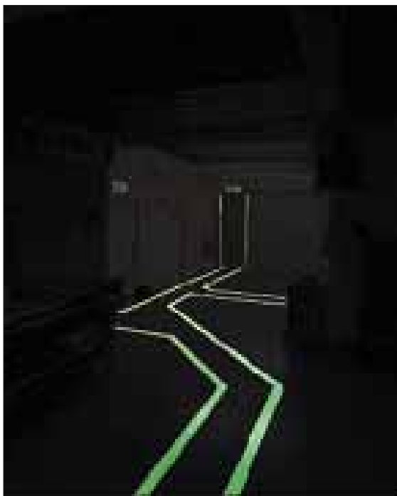
Figure 53: A 'way-guidance' system
