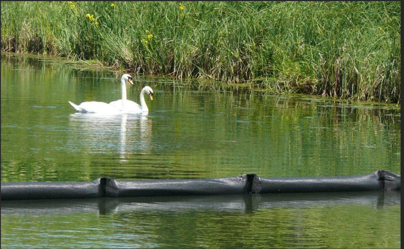
AquaticEngineering installed a flexible biomanipulation curtain across the mouth of the ponds to prevent the re-entry of fish and hold back the turbidity created by boats & operation of the locks.
