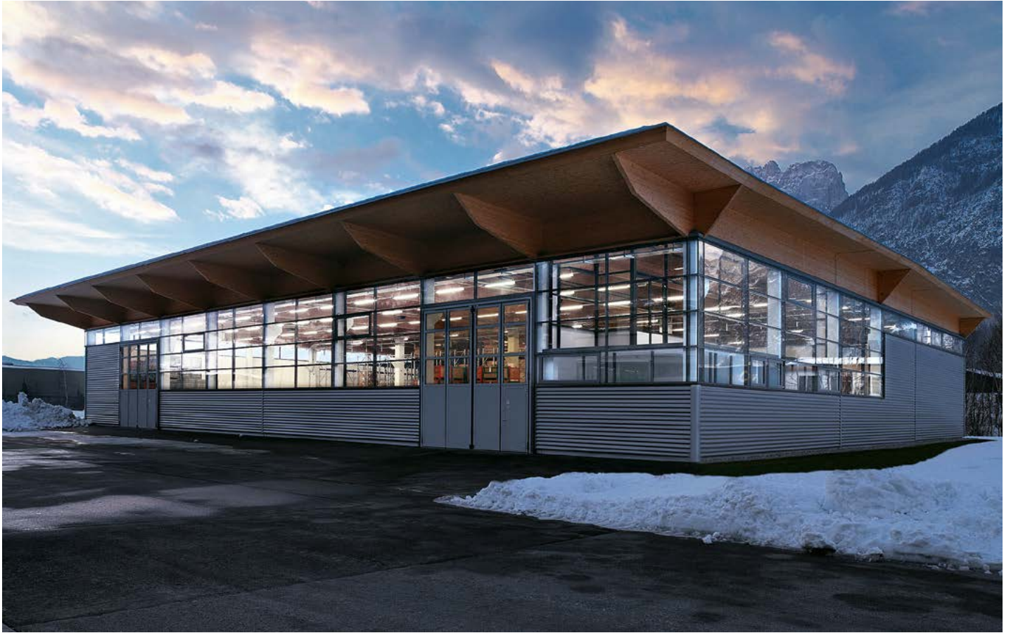
↑ IWT Innovative Water Technology GmbH, Lienz | AT Lighting solution: ZX2, CLARIS, ONLITE
