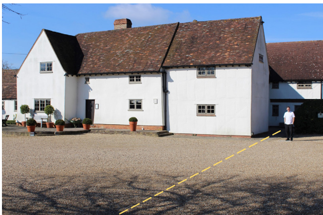
The drain run from The Plough to the main road is 30-40 metres long.
