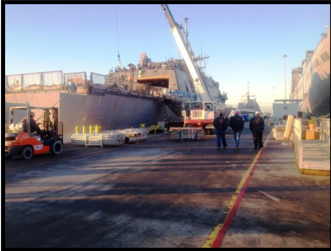
Start of superstructure scaffolding.
