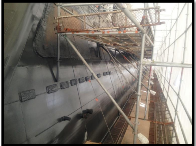
Steel & Aluminum substrates were abrasive blasted (Garnet & Copper Slag) and primed with epoxy.
