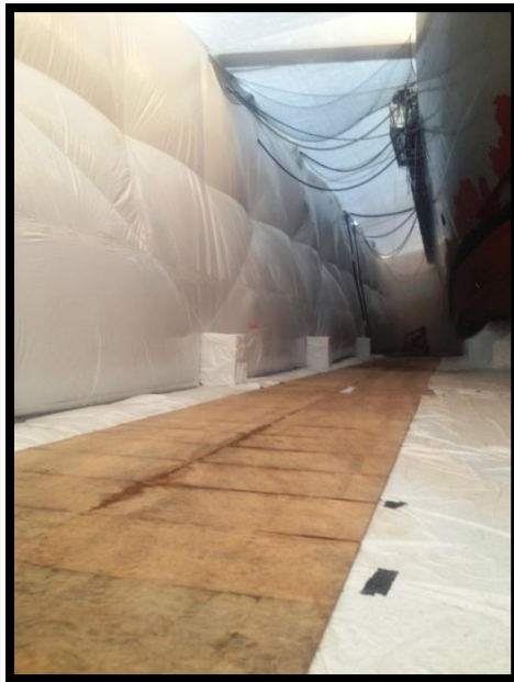
Encapsulation was completed & ready for surface preparation. The encapsulation was erected to a weather resistant degree due to the upcoming rain days which had been forecasted during the vessels availability.
