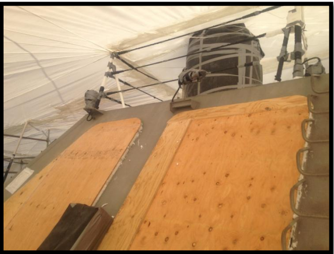
Installing protective covering on windows, vent openings, radar & appurtenances.
