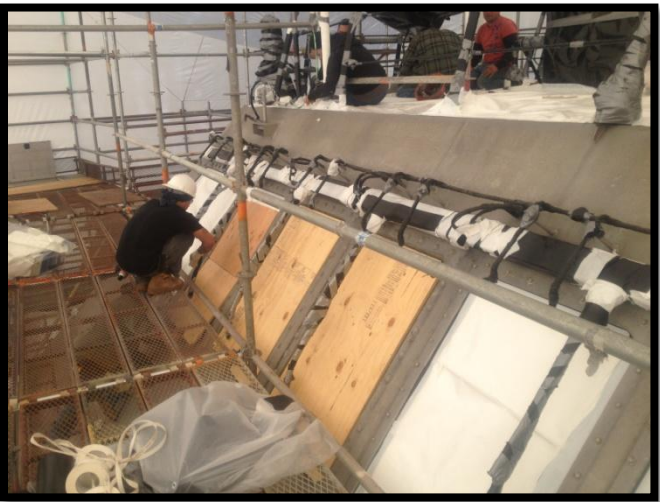
Installing protective covering on windows, vent openings, radar & appurtenances.
