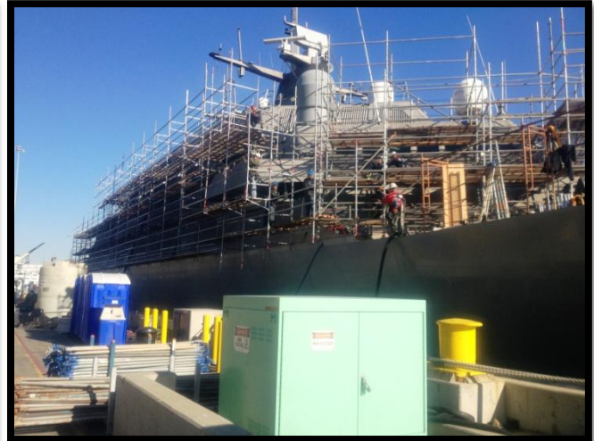
Superstructure scaffolding nearly completed pier side.
