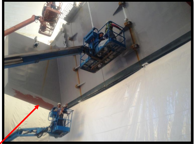
Encapsulation continues. Note existing coating failure areas.
