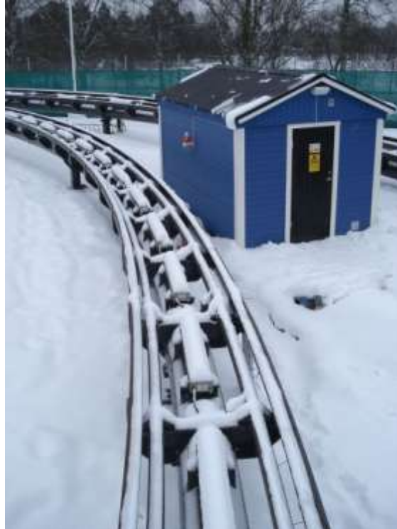
Figure 8. Linear motors in the acceleration ramp out from the station in Swedish winter weather.
