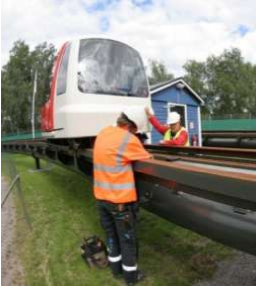
Figure 10. A full set of maintenance procedures has been developed that are verified during test track operation.
