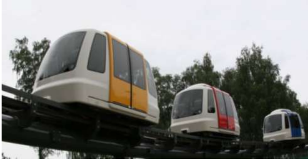
Figure 9. With the dynamic moving block control, vehicles can run with shorter distance between them at lower speeds.
