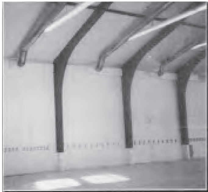
Figure 3.0 Solar Heat Air Duct (Alliance Church)
