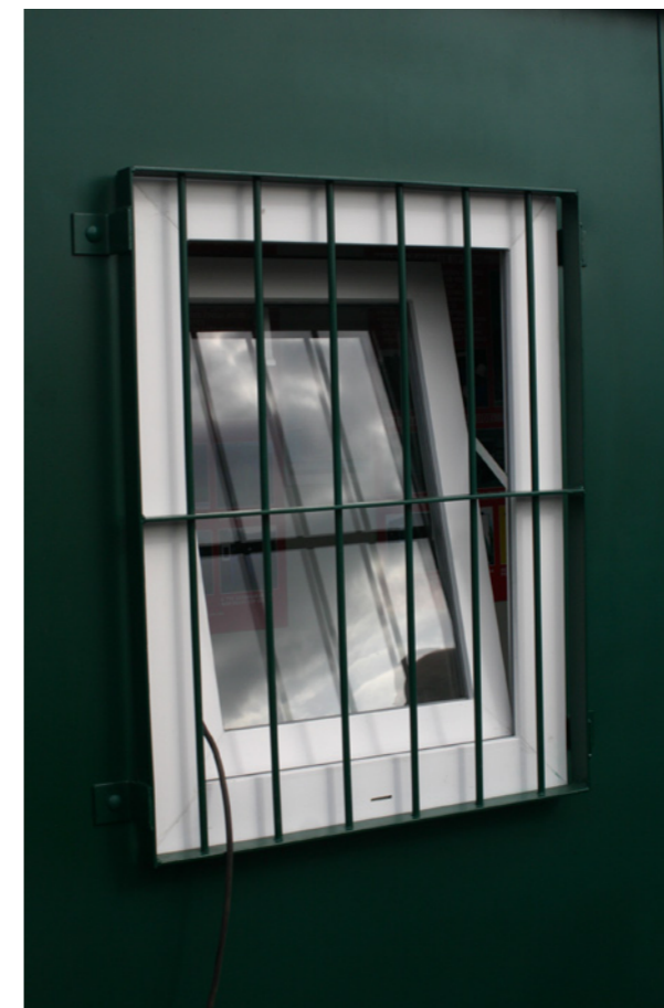
Window security grille cover
