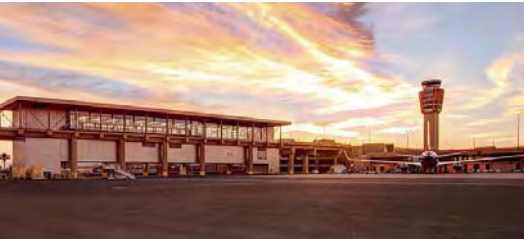
Work is scheduled to begin this year on a new concourse for Southwest Airlines at the Phoenix Sky Harbor International Airport.
