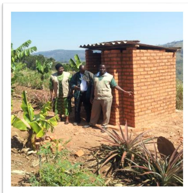
One of the 91 unsubsidized VIP latrines built
