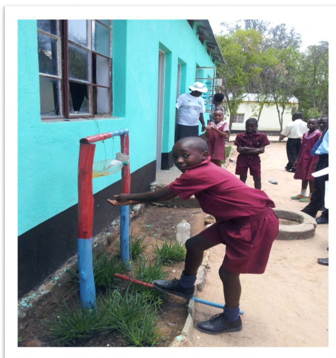
Wash Hand facilities outside all the classrooms
