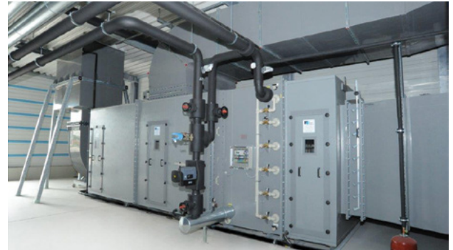
The Plastcon air handling system extracts valuable energy in the form of heat from the exhaust air, which can then be used for pre heating the incoming air steam.
