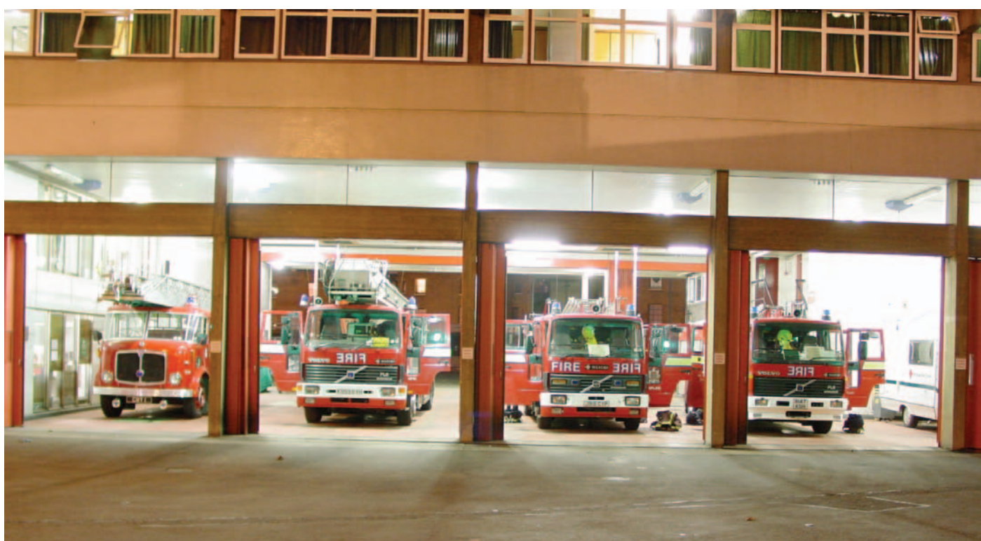
This night time image is of Paddington - one of London Fire Brigade's busiest fire stations. In view R to L are the stations two Pumps, and Aerial Ladder Platform. Far left is CBY 1, a 1964 AEC Merryweather Turntable Ladder, part of the LFB's historic collection which on this occasion was being temporarily housed at Paddington.
