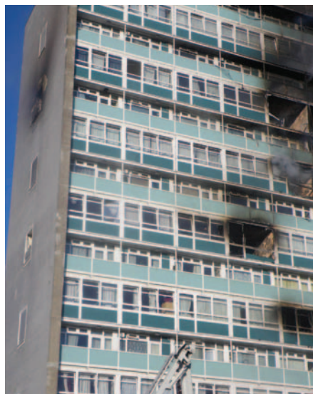
Camberwell high rise fire. Image courtesy London Fire Brigade
