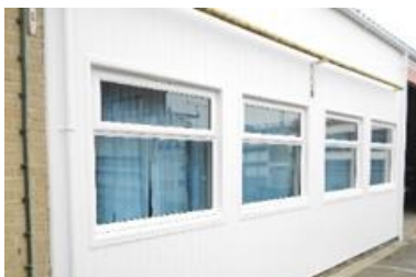
Yeovil Fire Station (After)
