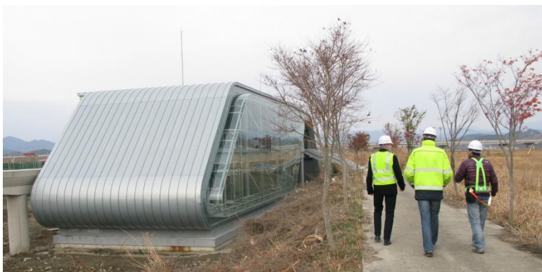
Station Two is near to completion
