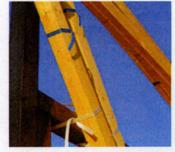
The trusses should be secured to the lorry by banding. This does NOT replace the need for the lorry driver to apply ratchet straps, but is for holding the trusses when the lorry/trailer is stationary; both in the suppliers yard and the customers site.
