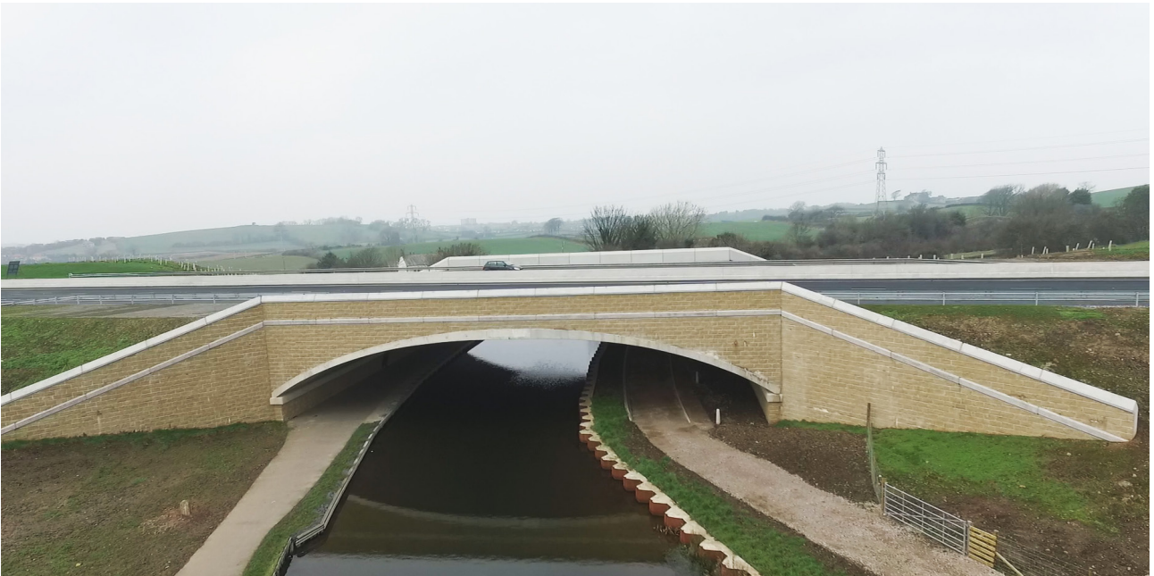
Heysham to M6 Link - Milestone Canal Bridge(654BI) (asset BEBO® Arch T94S - Span 28.651m - Rise 3.213m)
