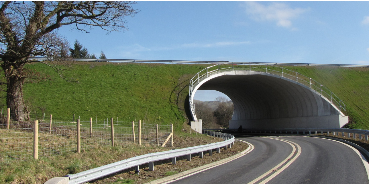
A470 Cwmbach to Newbridge -on-Wye- Red House Bridge (asset BEBO® Arch E15.5Mt/5 - Span 15.5m - Rise 5.6m)
