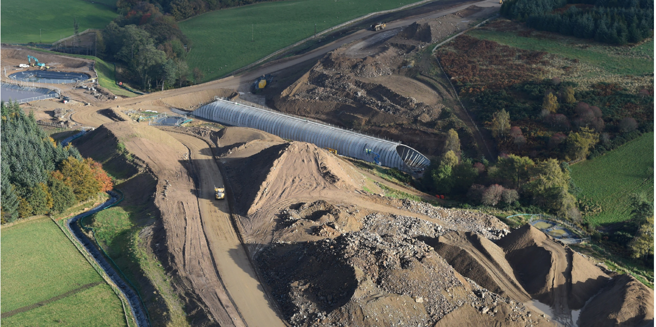
Aberdeen Western Peripheral Route PS02 and PS41A (asset BEBO® Arch C42T/9 - Span 12.802m - Rise 8.026m)
