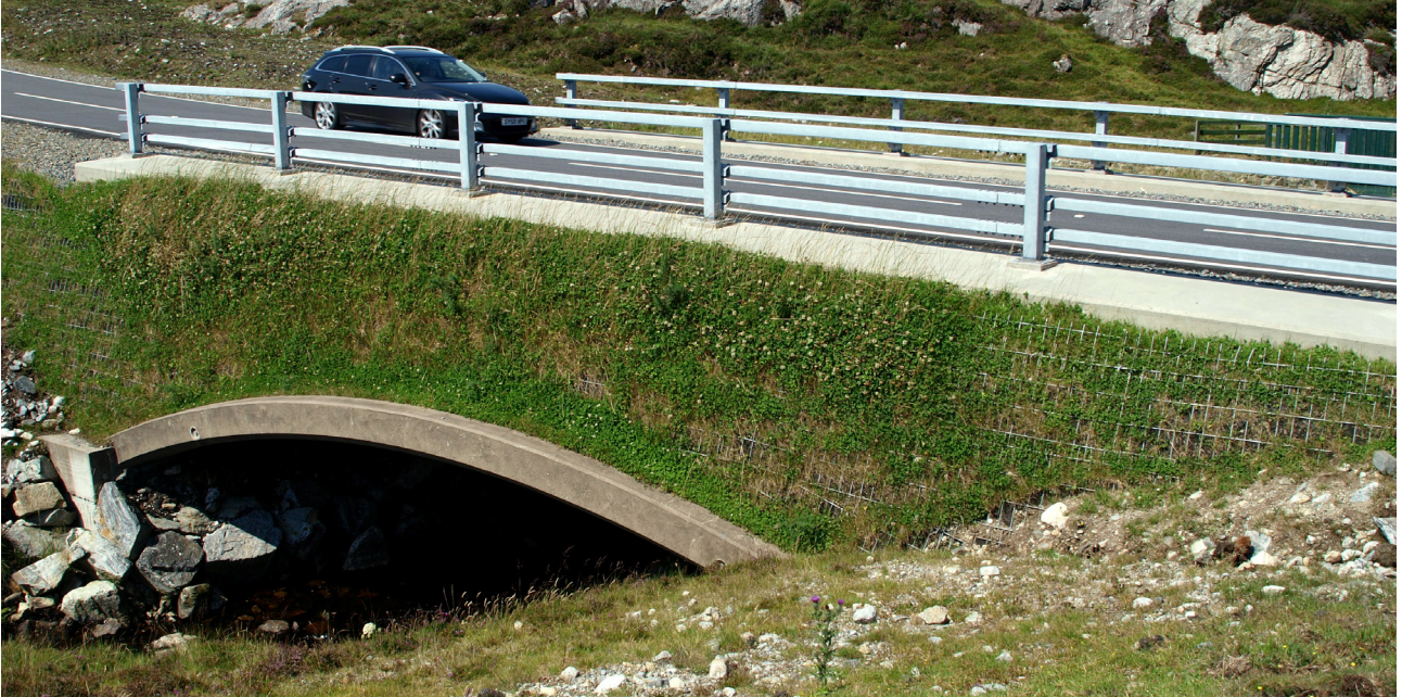
Stornaway - Gisla Bridge (asset BEBO® Arch T36 - Span 12.108m - Rise 1.382m)
