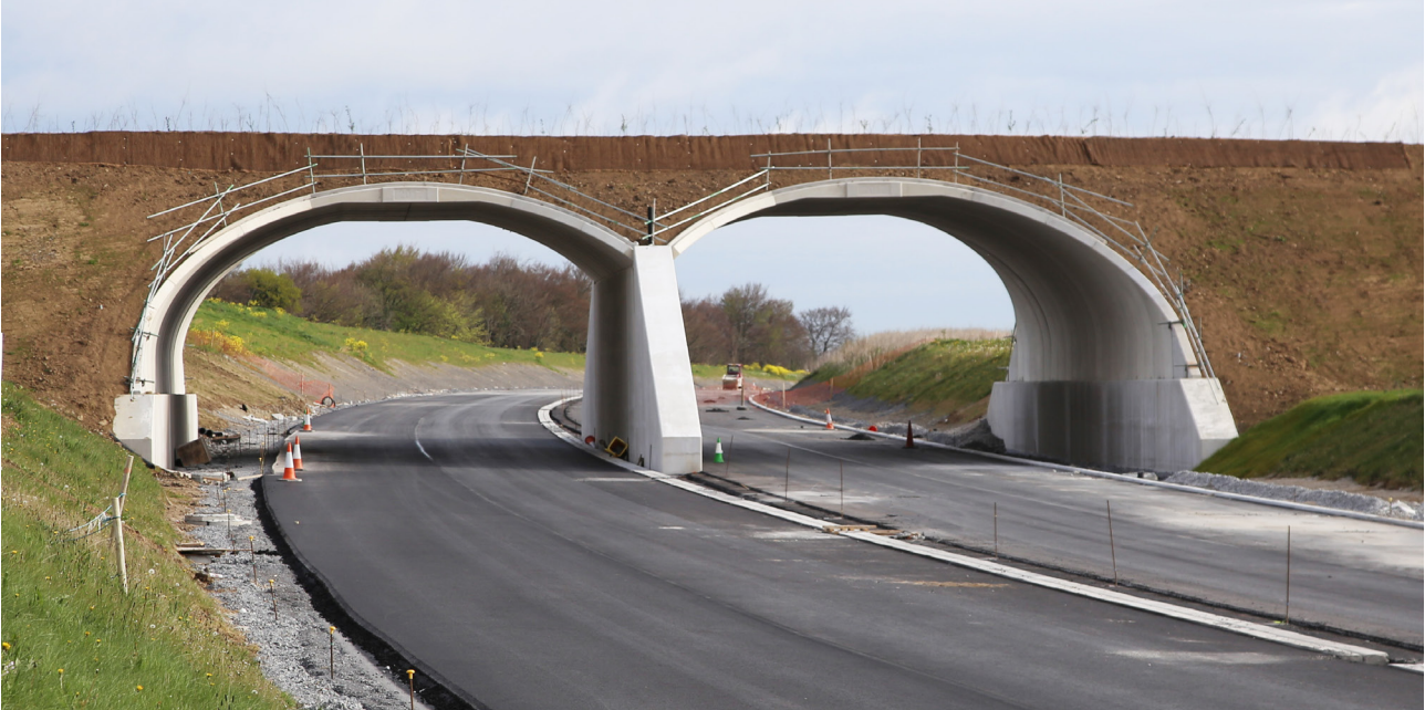
N17/N18 - Gort to Tuam - OB241 Coole Green Accommodation Overbridge (asset BEBO® Twin Arch E15.5mT - Span 14.3m - Rise 5.9m)
