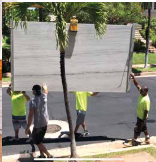
Tim Lloyd Construction crew uses a small crane to move a 60-square-foot slab of quartzite into the home site. PHOTO COURTESY TIM LLOYD CONSTRUCTION
