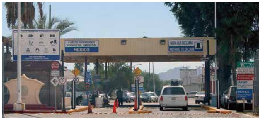
Construction of a border wall has begun at Lukeville, Ariz.
