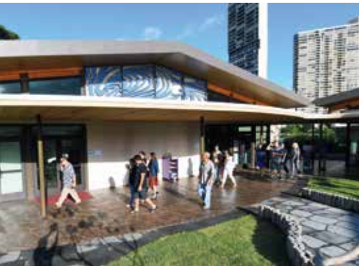
Allied Builders System completed Iolani School's K-1 Community in time for the 2019-2020 school year.
