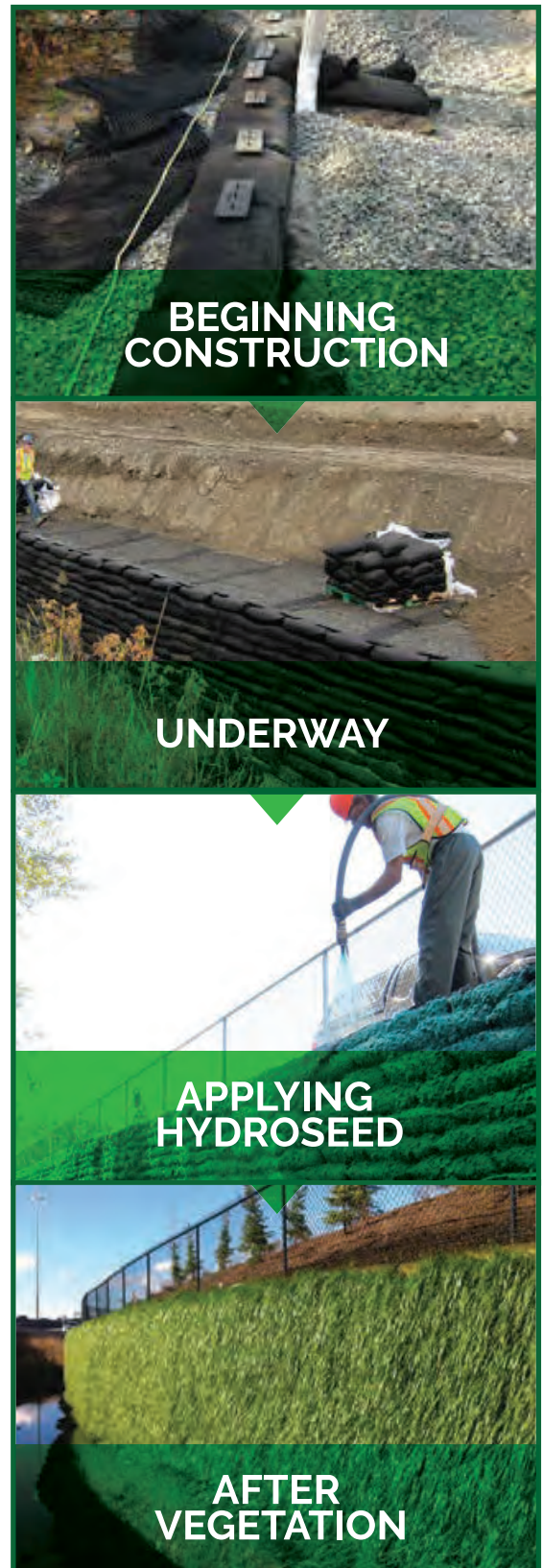
5m (16ft) tall commercial retaining wall
