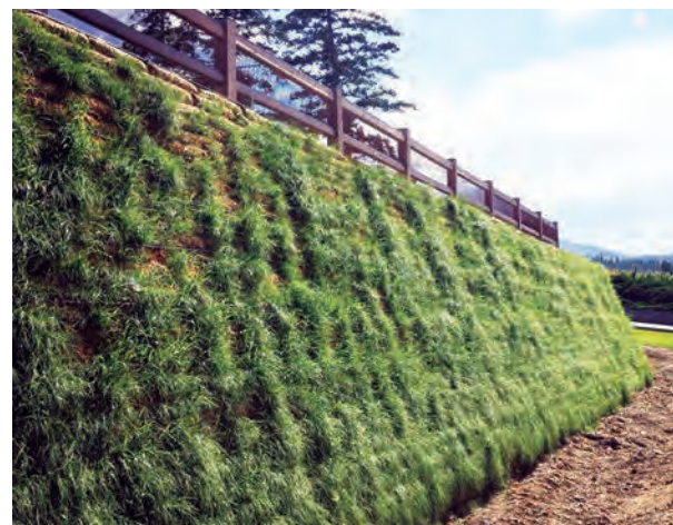
5m (16ft) tall landscape retaining wall
