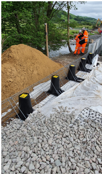
Black Bridge Machynlleth Supplied asset BaFix™ 70 and Sleeve-It
