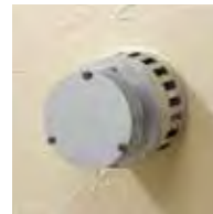
Balanced Flue (No chimney required)
