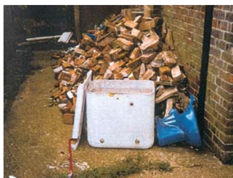
Figure 12 Asbestos cement tank
