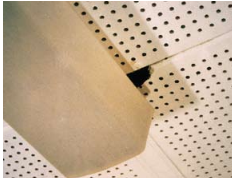
Figure 6 Perforated AIB ceiling tiles
