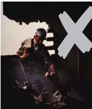
Figure 39 A workman has broken through a brick wall. This disturbed a previously hidden lining of AIB.
