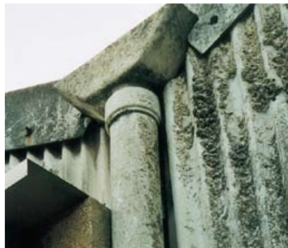
Figure 15 Asbestos cement drainpipe
