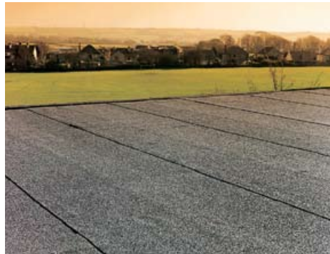
Figure 13 Built-up bituminous roofing containing asbestos
