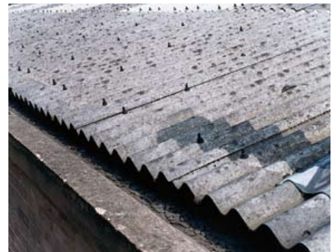
Figure 7 Asbestos cement roof
