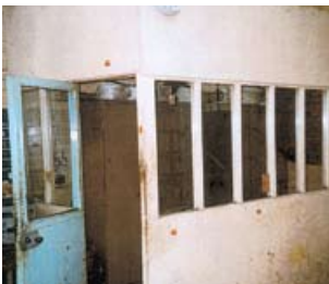
Figure 28 An office made from AIB
