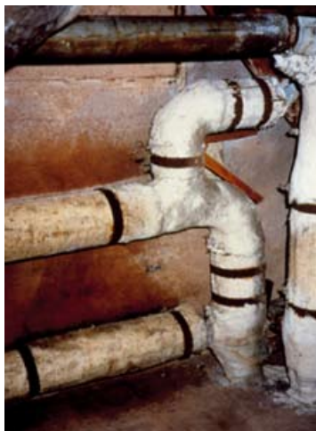
Figure 23 Asbestos pipe lagging
