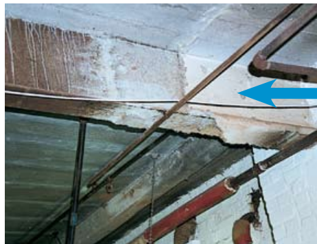
Figure 27 Sprayed 'limpet' coating which has been partly removed
