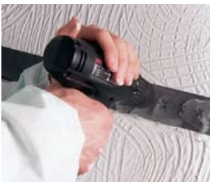
Figure 50 Drilling through paste
