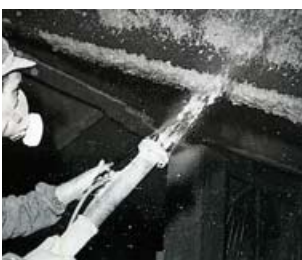
Figure 36 Installing a sprayed 'limpet' coating
