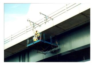
The inner portion of the Suspended Access Platform is suspended from the existing bridge runway beams via beam trolleys whilst the outer portion is suspended from the mobile davits. The modular Steel Truss Frame platform has a working area of 2.44M X 3M. Access to and from the platform is via secured ladder and inertia reel safety devise.
