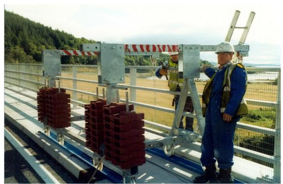
ALPS Delta Suspension Beam with 1M reach; 1.2M rear of fulcrum & raised to clear the parapet is fitted with 30 X 25Kg (750Kg) captive weights on each beam ensuring a 3-1 coefficient of safety. The suspension beams run in free laid tracks and are propelled and restrained by hand operated wire rope winches.
