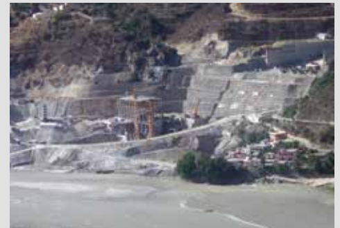
Alakanada Dam, India
