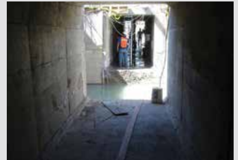
Ensenada International Terminal Tunnel, Mexico
