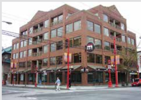
Channel M Building, Vancouver, Canada
