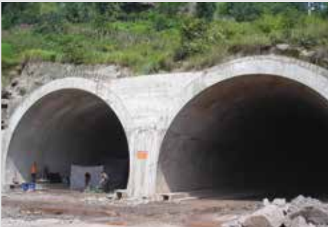
Yunnan Shuima Tunnels, China
