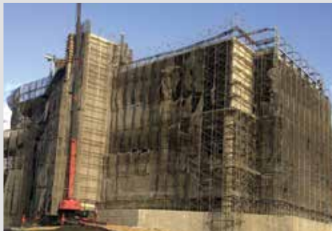
Tung Ho Steel Plant, Taiwan
